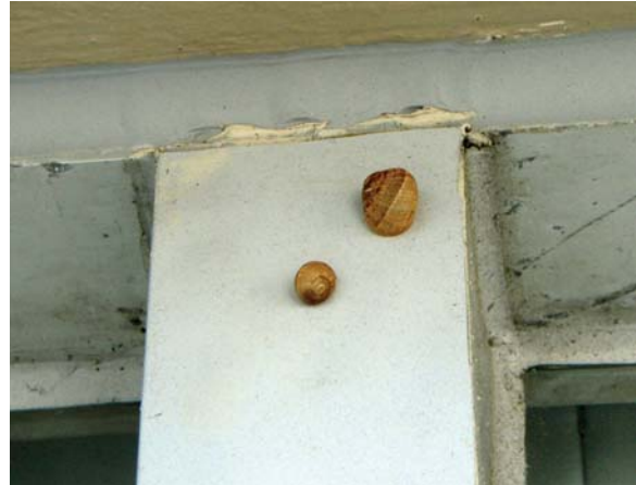
Above: Silicone tape flashing on a condominium in San Francisco.
